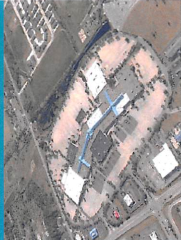
ILLUSTRATIVE MASSING SHOWS POTENTIAL TRANSFORMATION TO A VIBRANT, WALKABLE & MIXED-USE DISTRICT FROM AN AUTO-ORIENTED SINGLE-USE MALL (BELOW).
