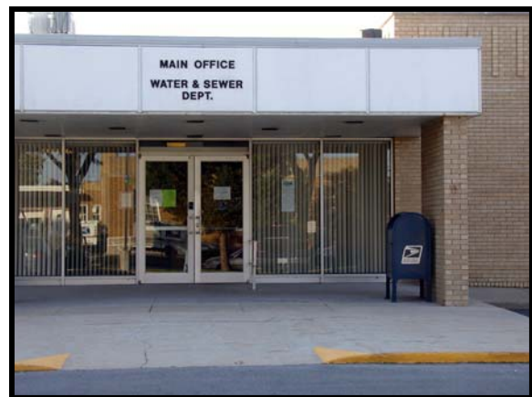
The Village of Bradley’s Water & Sewer Department
