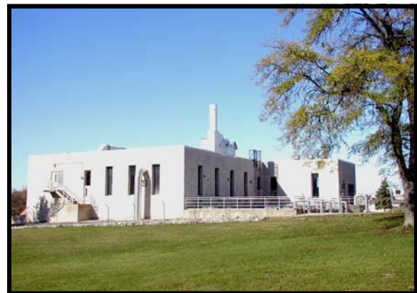
The KRMA's sewage treatment plant, on the Kankakee River.
